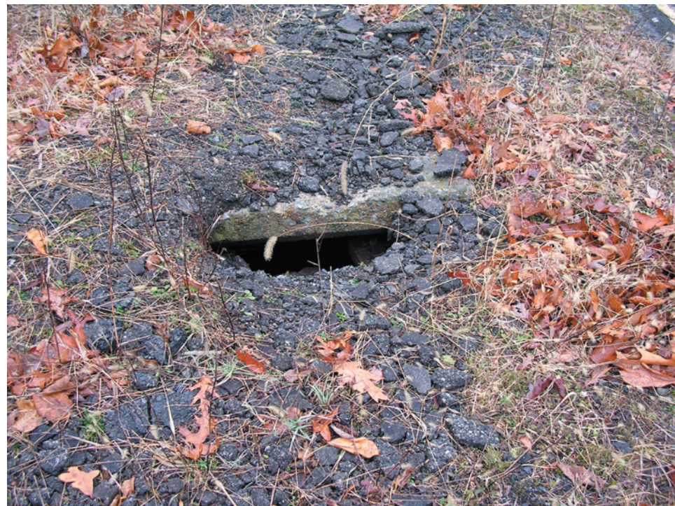
Culvert blocked by roadway debris.
