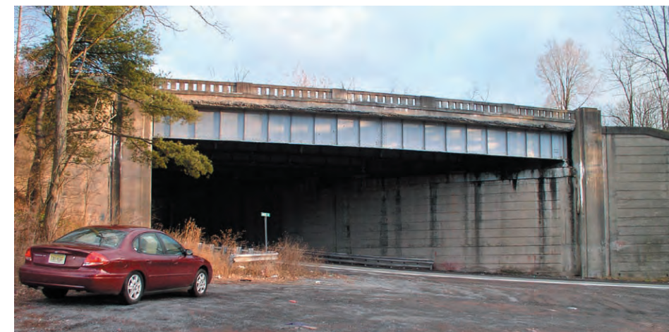
Conditions of the above structure prior to demolition.
