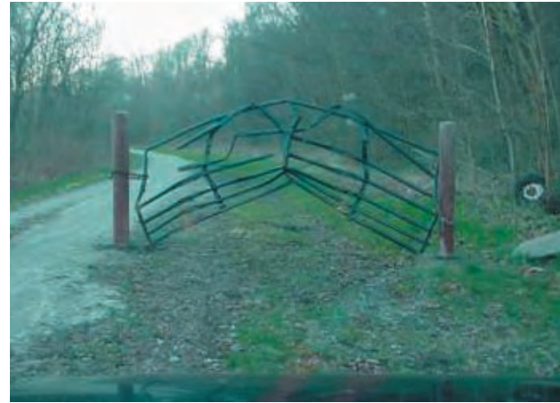
Damaged livestock type gate.
