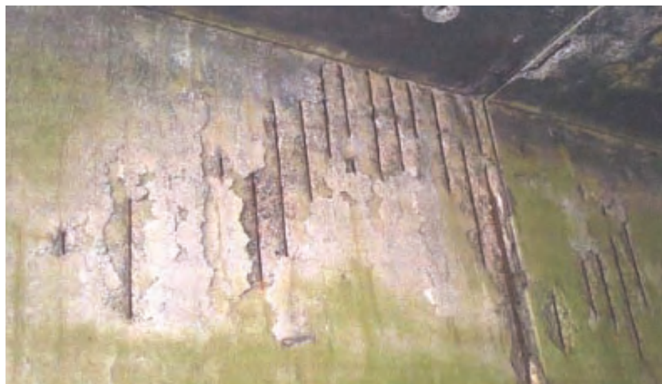
Delamination and Spalling.
