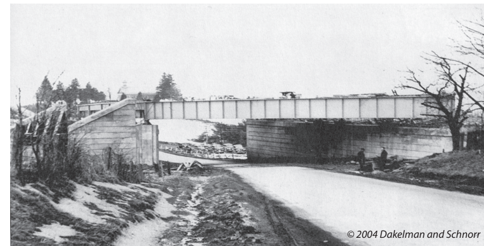
The structure carrying the Turnpike over Route 30 at breezewood while under construction.
