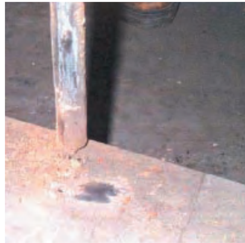
Corroded and broken support rod
