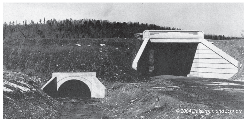
A small concrete arch culvert and a T-beam bridge between Ray's Hill and Sideling Hill Tunnels.
