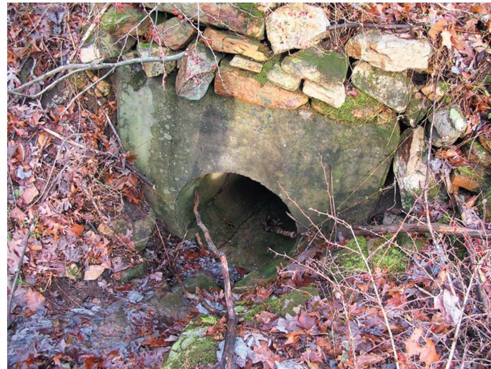
Culvert exhibiting channel debris.
