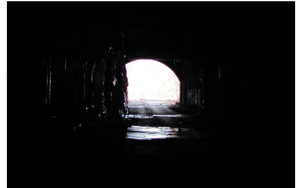
Peering out from inside Sideling Hill Tunnel.
