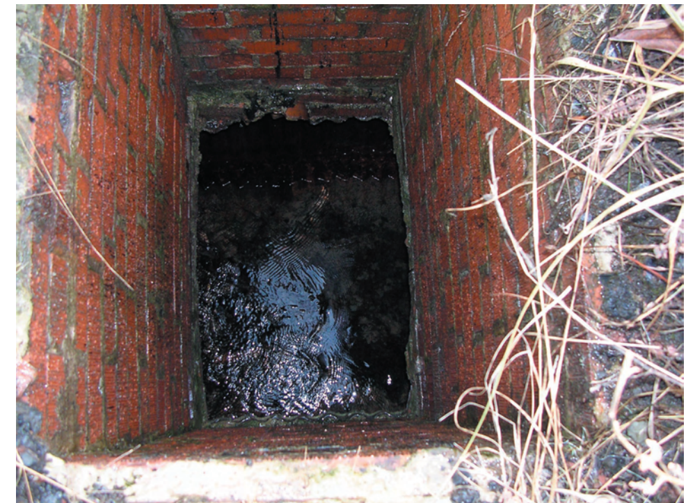
An open drainage inlet.
