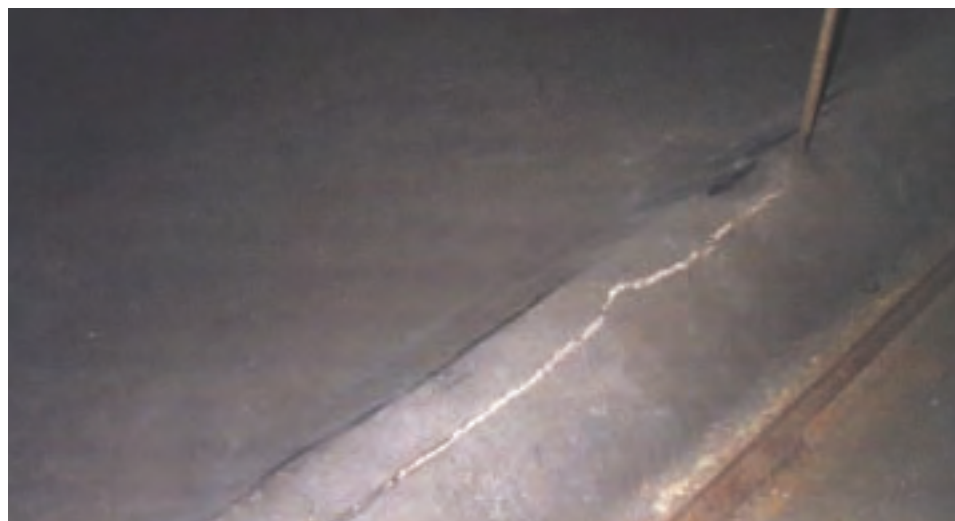
A portion of cracked ceiling in Ray's Hill Tunnel
