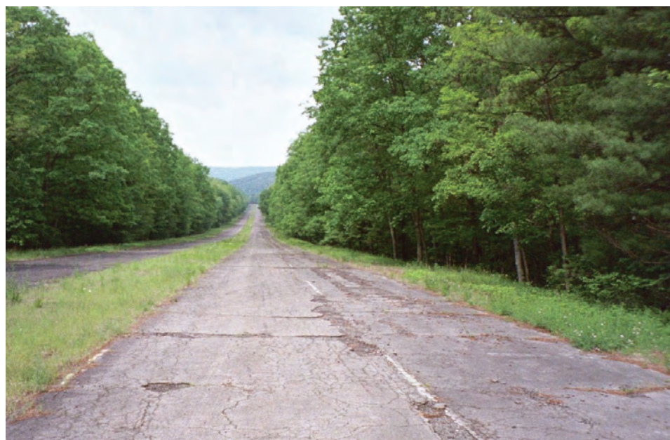
Examples of raveling and reflection cracking along the same stretch of highway.
