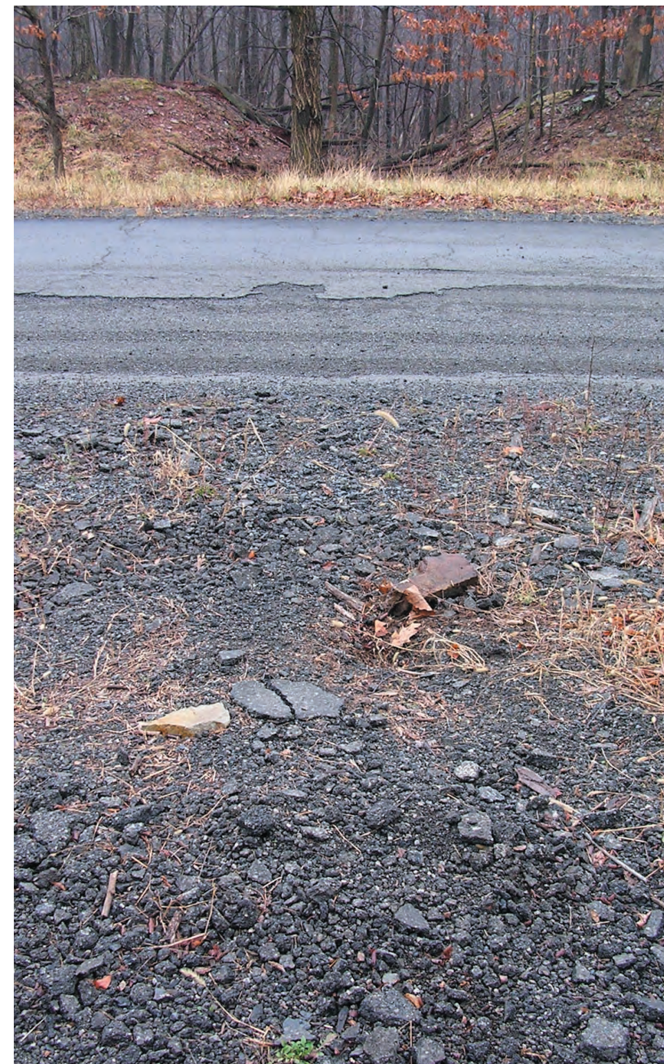
A detailed view of current pavement distress.
