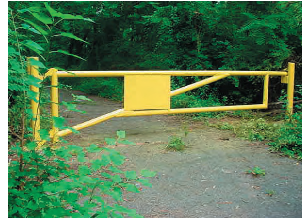
Newly installed trail gate.
