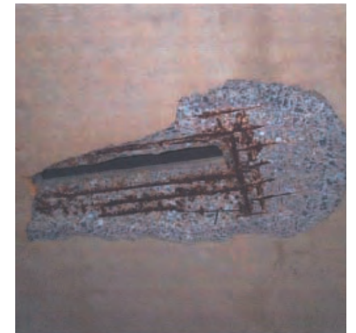
Ceiling spall and exposed rebar around air vent
