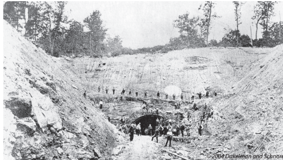
© 2004 Dakelman and Schnorr Eastern portal of Ray's Hill Tunnel during construction
