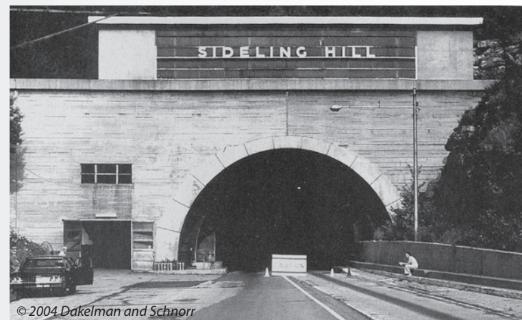
Sideling Hill Tunnel shortly after its closure
