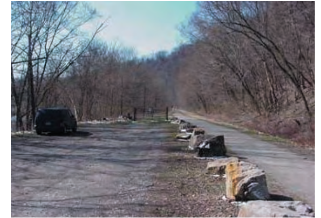
Boulders placed to create barrier.
