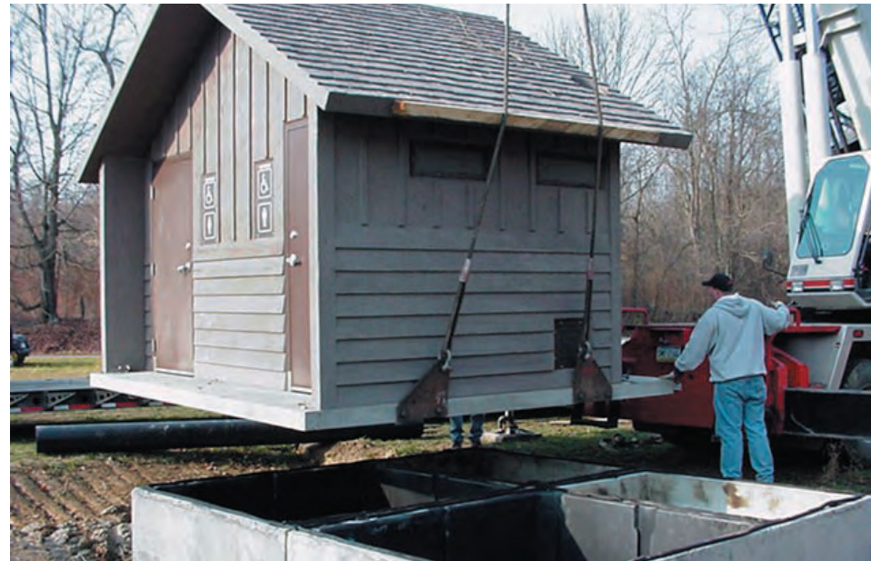
Sweet Smelling Toilet being installed.
