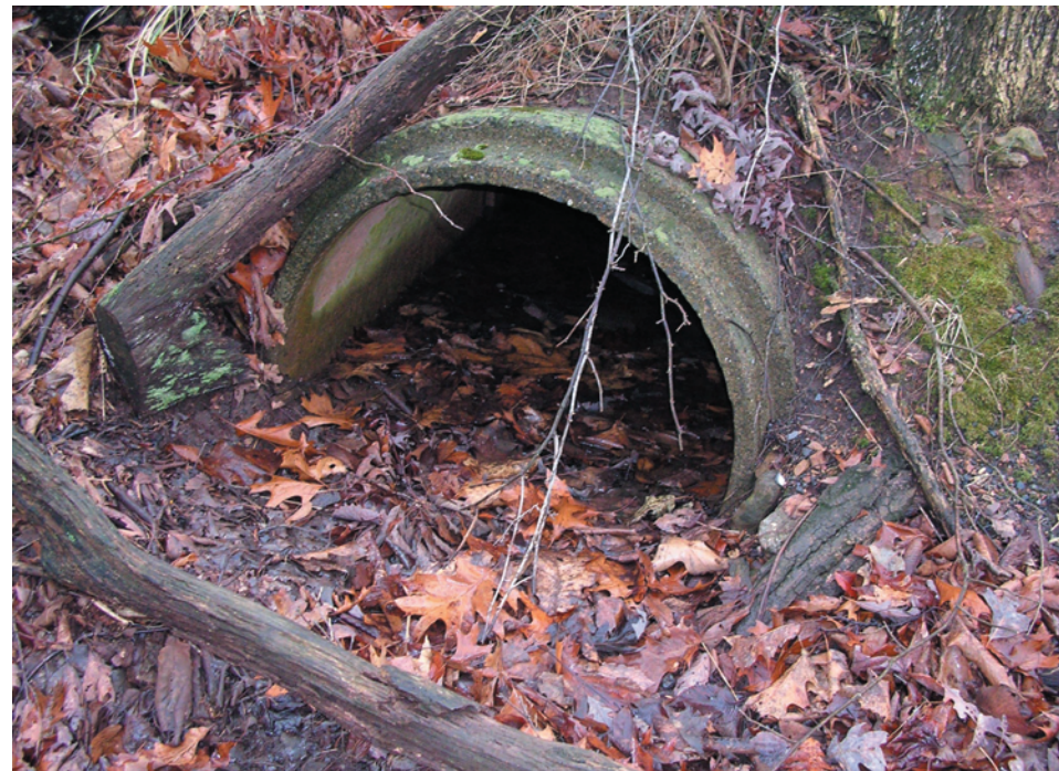
Another example of a drainage culvert choked by debris.
