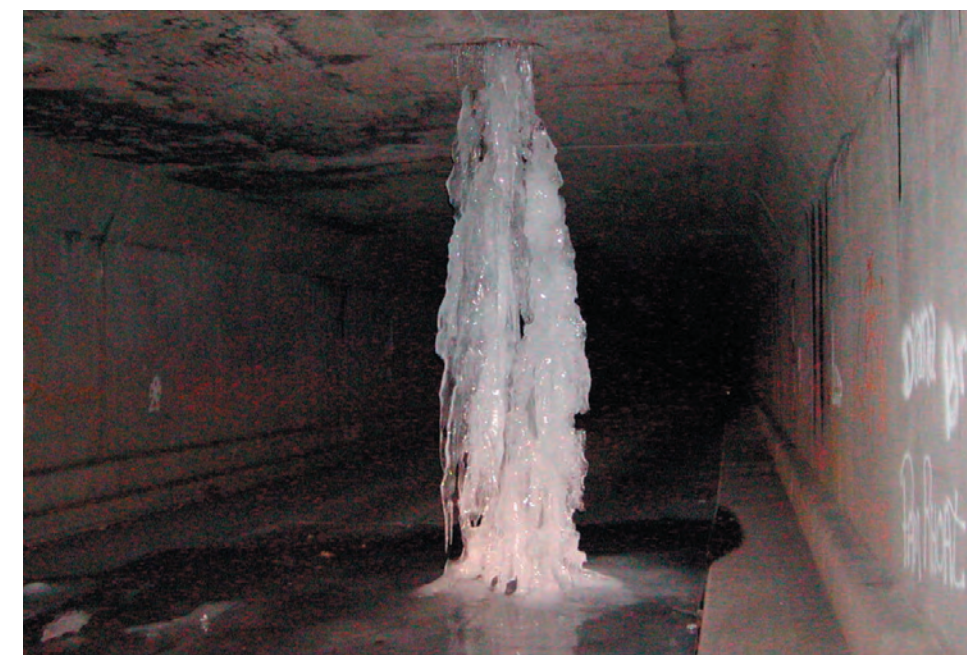
Large amounts of ice can form during the winter months obstructing the tunnels.
