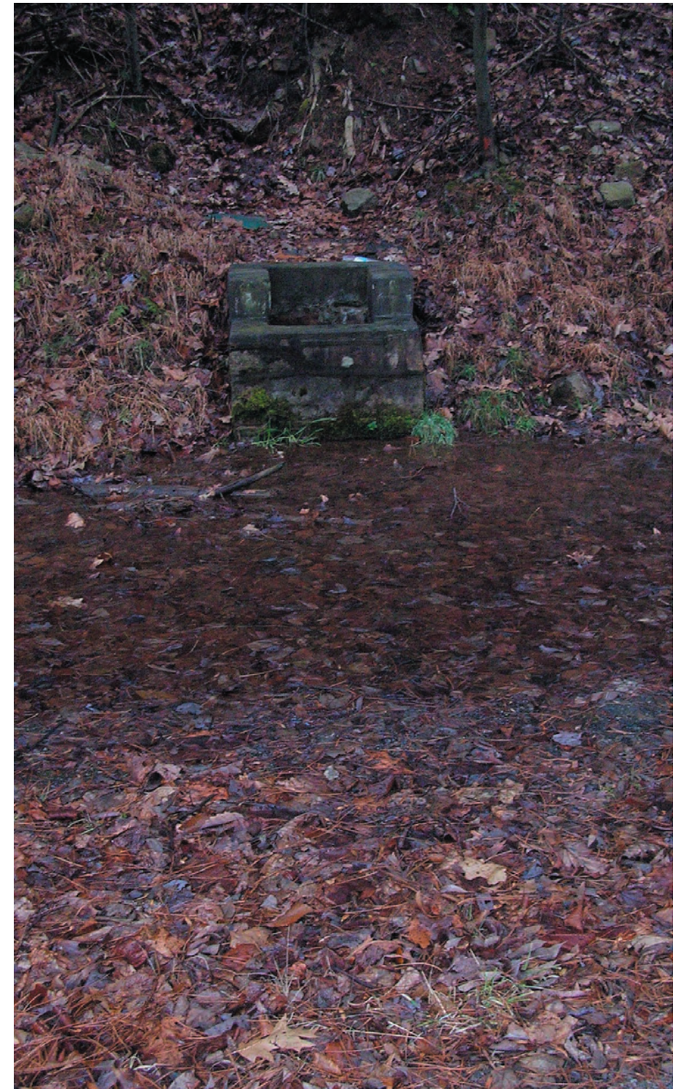
A spring area exhibiting poor drainage.
